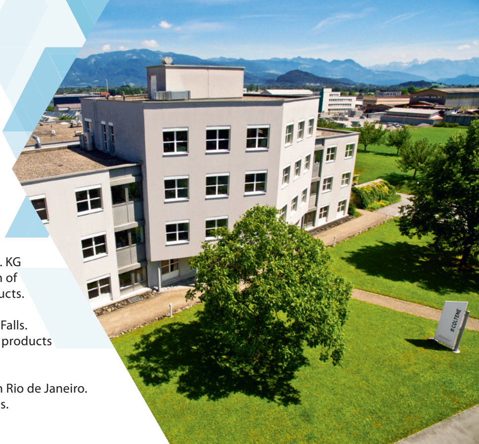
COLTENE Headquarter, Altstätten / Switzerland
